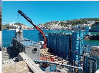
Ponza: enhancement of wastewater treatment plant
