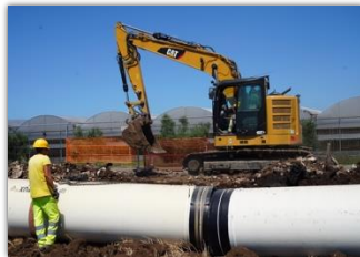
Acqualatina: Sardellone pipeline doubling
